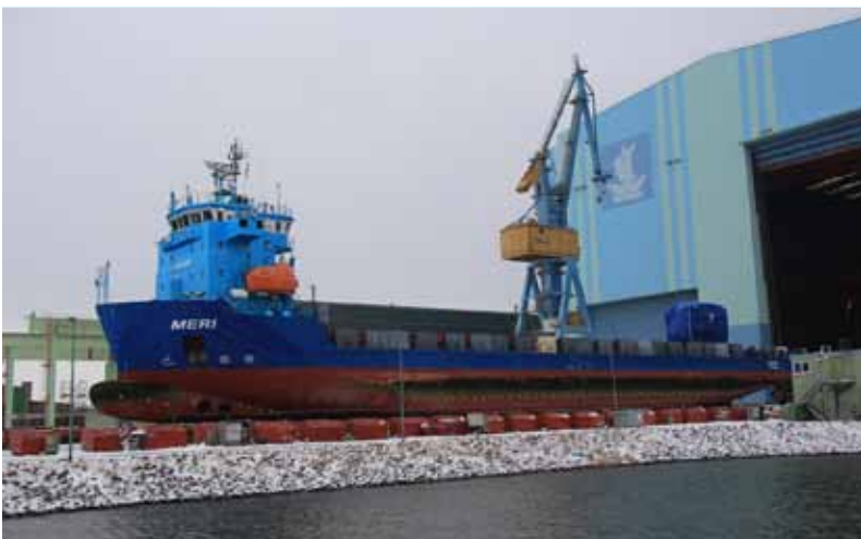
Sometimes it is not possible to bring cargo to the quay side. In this case it was possible to lift the vessel and skid mv MERI to the assembly hall and perform loadout in the hall with overhead cranes.
