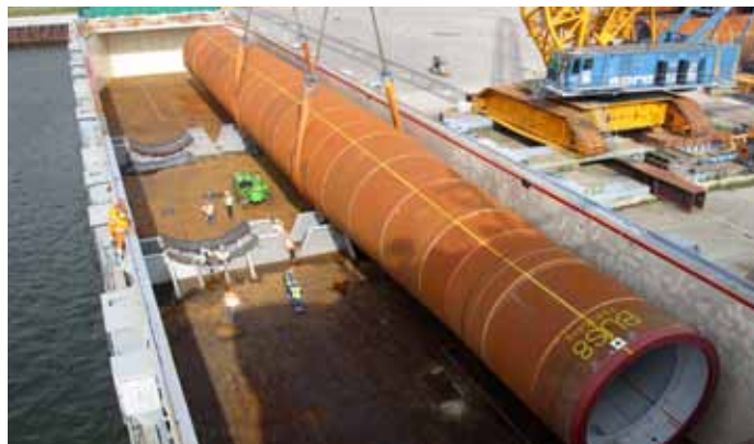
Gemini monopiles North Sea Sea transport, engineering
