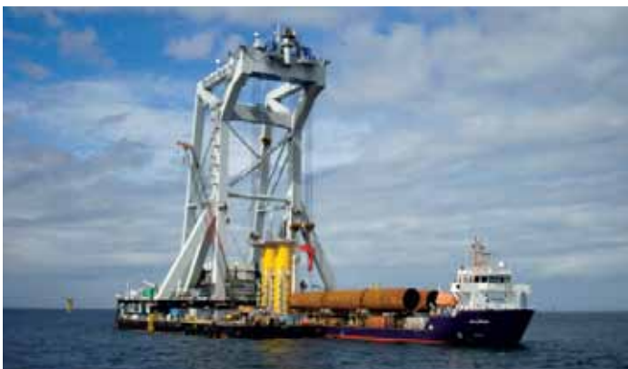
Windmill foundations Holland / Offshore site, UK East coast Sea transport
